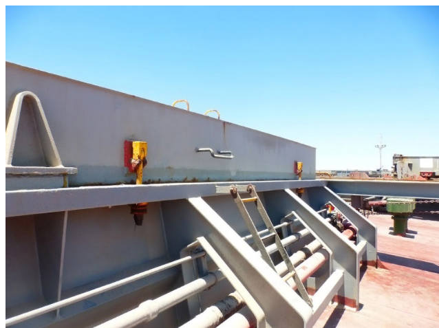
Figure 26: Maintenance of the hatch cover structure
