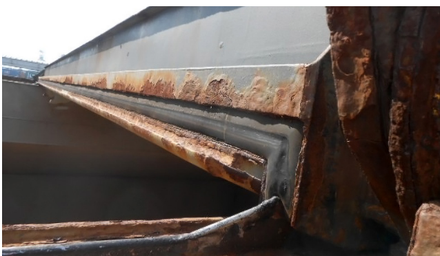
Figure 27: Maintenance of hatch cross joints
