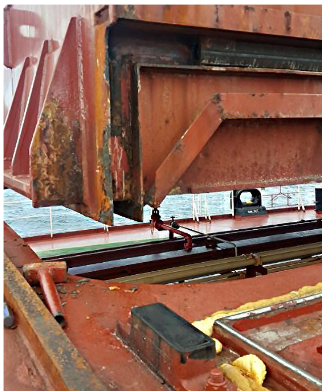
Figure 36: Maintenance of gasket channel
