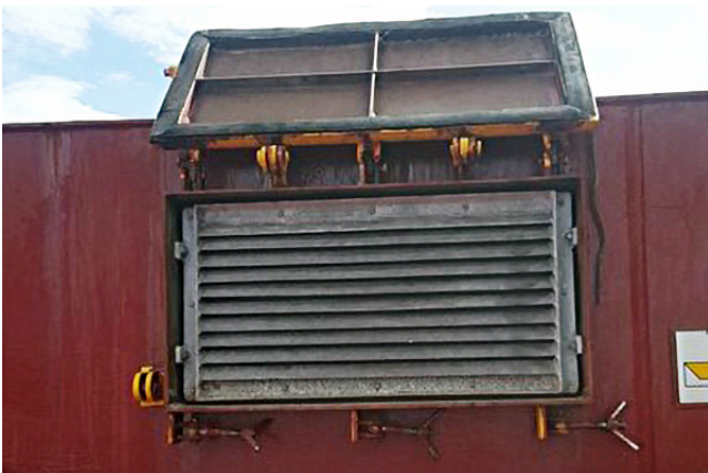
Figure 42 (a and b): Maintenance of rubber seals on access hatches and ventilators
