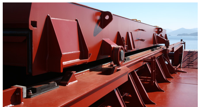
Figure 31: Maintenance of hatch wheels and trackways
