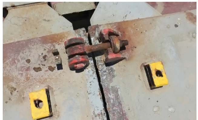
Figure 20: Inspect condition of cleats and panel for distortion
