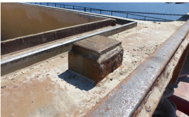
Figure 30: Maintenance of the landing pads
