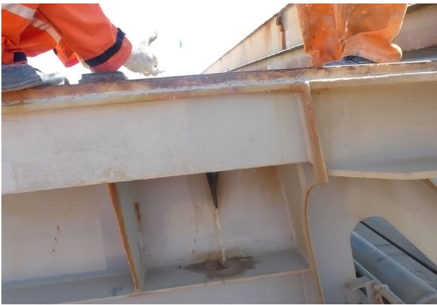
Figure 29: Maintenance of hatch coamings
