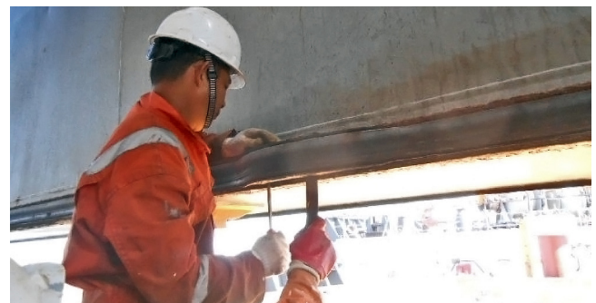
Figure 34: Replacement of the entire length of aged gasket
