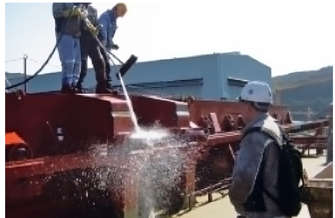
Figure 18: Water hose leak detection test
